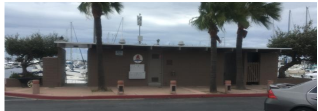
Existing 1960's Restroom, scheduled to be replaced
