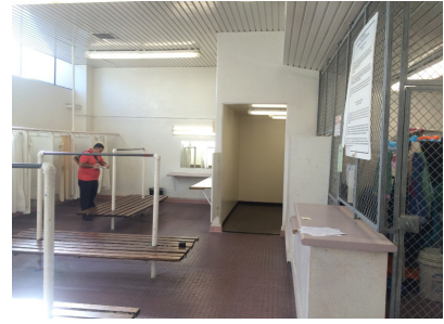
Locker Rm Before Renovation
