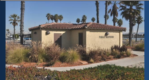
72nd Place Beach Restroom, Long Beach
