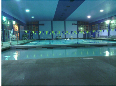
Indoor Pool Before Renovation
