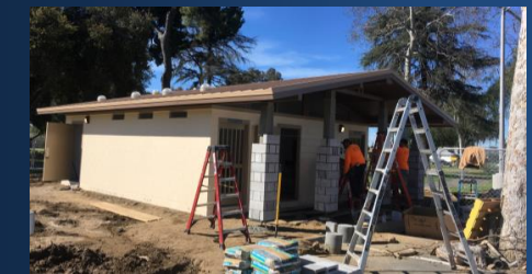
De Anza Park Restroom, Ontario
