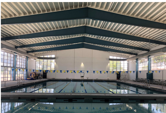
After: New Ceiling Structure, New Lighting,
