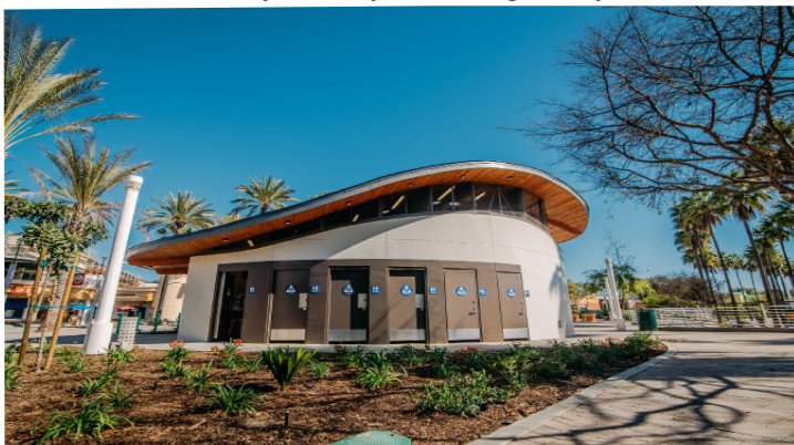
Queensway Beach Restroom
