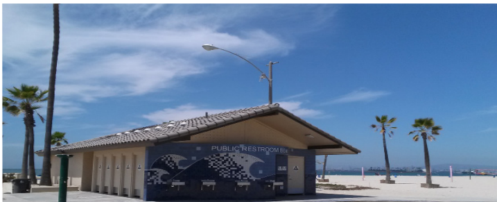
Granada Ave. Beach Restroom & Concession Renovation
