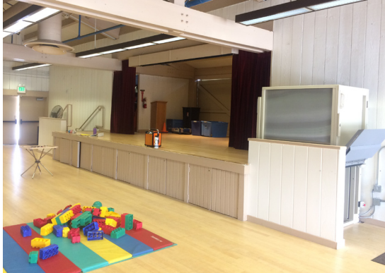
New access lift and accessible stair retrofit
