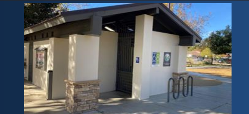
Sumac Park Restroom, Agoura Hills
