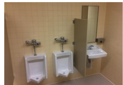
new accessible restroom
