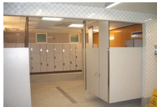
New Dressing Stalls and Floor Drains
